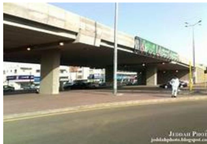
Picture showing overhead bridge in Ado-Ekiti
